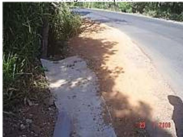
Trinca na Sarjeta Executada
